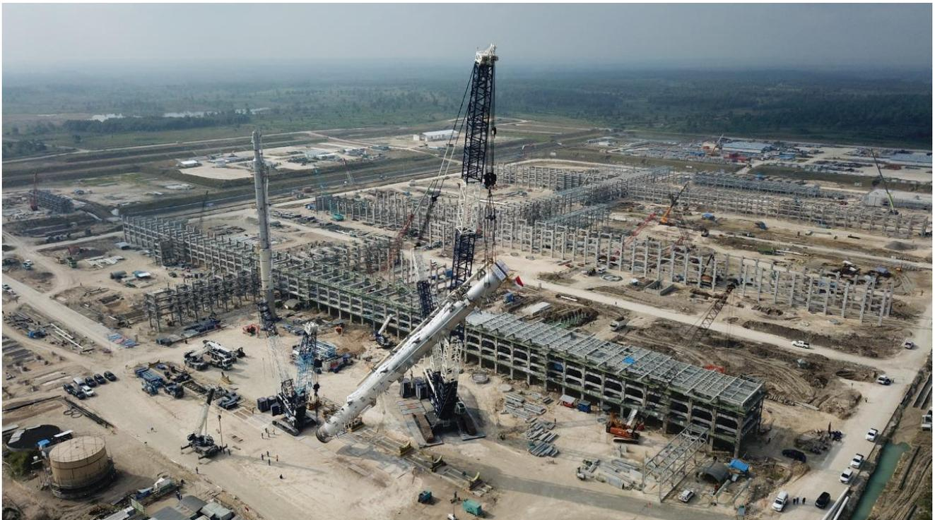
Proses *Heavy Lifting* Absorber 508T Proyek JTB *Drone View*
